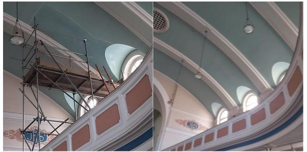
You can see the scaffold has been and gone, the large hole from water damage has been repaired and the lime plaster including breathable paint to keep in line with the traditional methods and conservation rules. A lovely piece of workmanship using the traditional methods.
